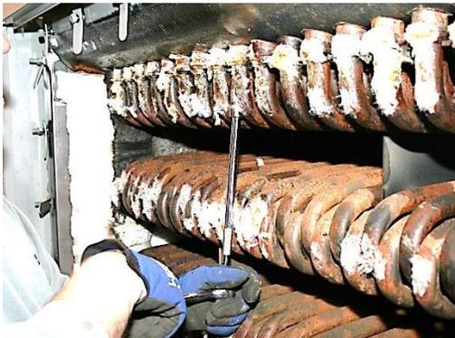
2. **Remove upper tube clamps.** Follow the same procedure as step 1 above.
