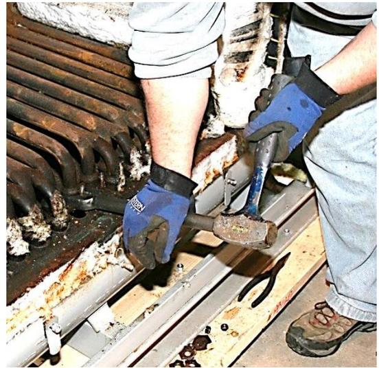
8. **Pull inner row tube-ends.** Repeat the procedure in steps 4 through 7 to remove inner tube(s).
