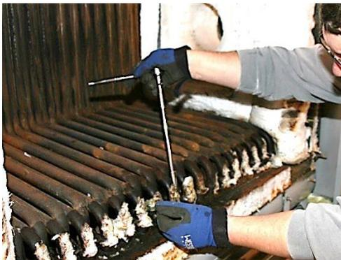
1. **Remove lower tube clamps.** On most models a stud and clamp are required over the tube flange. Remove the retaining nut and clamp before attempting to remove tube(s). To facilitate removal, you may need to soak with a good penetrating fluid.
