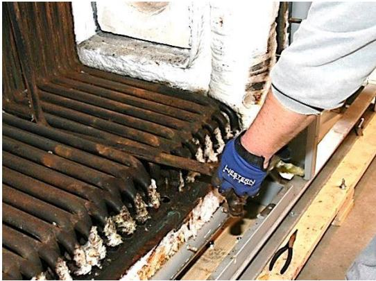
7. **Remove outer row tube.** Remove the tube and repeat with the other outer row tubes to gain access to rear tube, two adjacent outer tubes must be removed first to access the inner tube removal.
