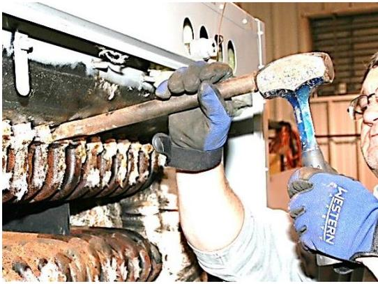
6. **Pull upper tube-end.** Repeat the procedure to pull the tube-end of the same tube from the upper header.
