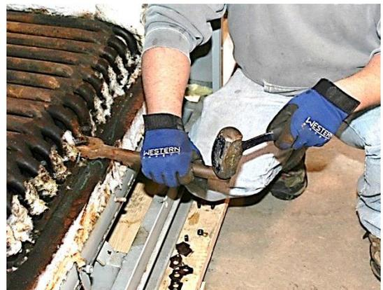
5. **Clear tube-end from the header.** Continue driving wedge under and levering flange up until it pops the end of the tube free from the hole in the header.
