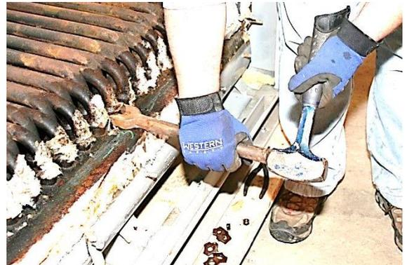
4. **Pull lower tube-end (outer row of tubes).** Wedge the tube puller under the flange of the tube. Drive the tube puller with several blows with a hammer on the end of handle. Alternate with downward blows to lift tube-end. Hold the leverage and repeat to drive the wedge further.
